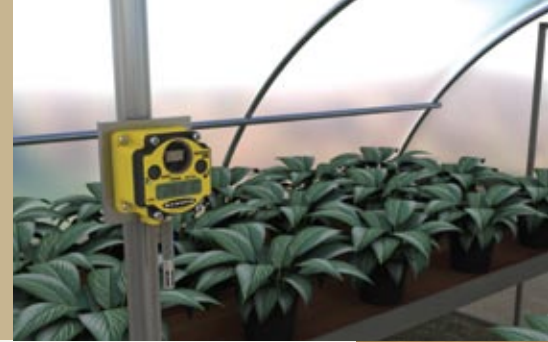
Greenhouse Temperature and Humidity Monitoring
