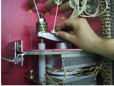
Handling of indicating spring and mounting clamp
