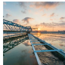
Waste water treatment plants
